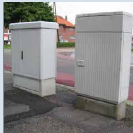
XDSL cabinet Next to copper cross connect
