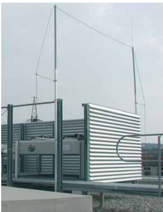
Fig. 5.1.8.14 Isolated air-termination system with DEHNiso-Combi
