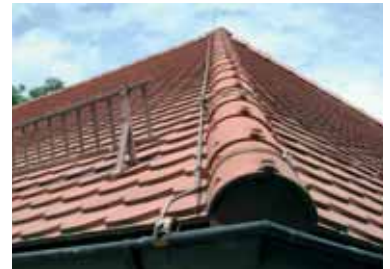
Fig. 5.2.2.1.3 Air-termination system with connection to the gutter
