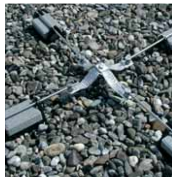
Fig. 5.4.1.1 Air-termination system – Compensation of expansion with bridging braid
