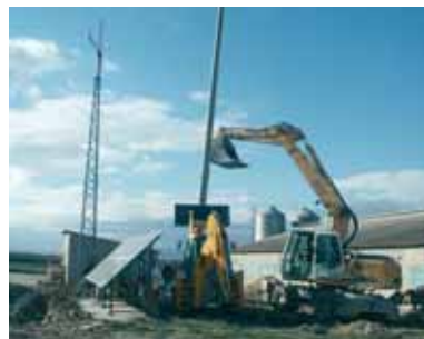
Fig. 5.1.8.9 Installation of a steel telescopic lightning protection mast
