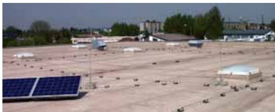
Fig. 5.1.3.3 Use of air-termination rods
