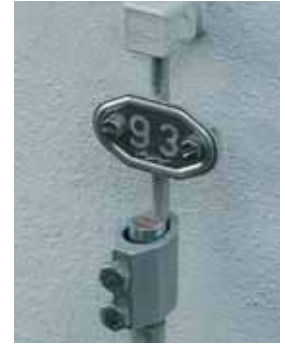
Fig. 5.2.2.3.1 Measuring point with number plate
