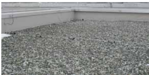
Fig. 5.1.3.2 Air-termination system on a flat roof
