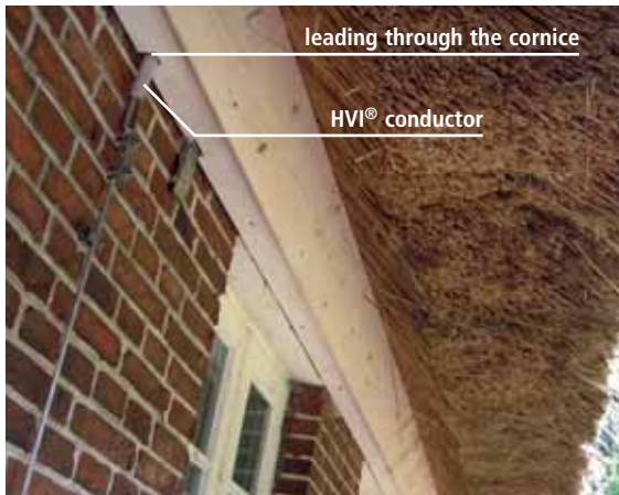
Fig. 5.1.5.7 HVI conductor led through the cornice plank
