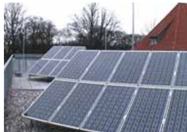
Fig. 5.1.8.6 Isolated air-termination system for photovoltaic system
