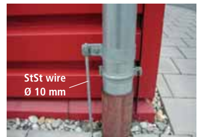
Fig. 5.2.2.1.4 Earthed downpipe
