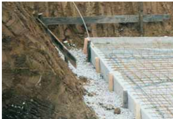
Fig. 5.5.2.4 Foundation earth electrode in use
