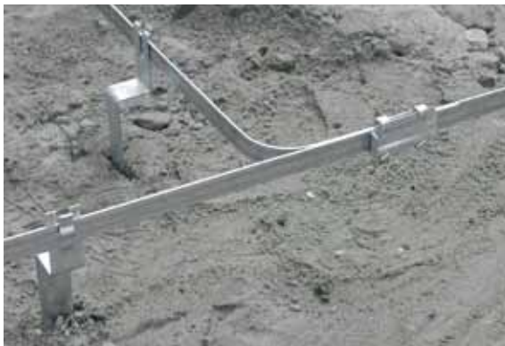
Fig. 5.5.2.3 Foundation earth electrode
