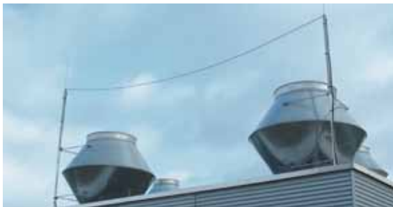
Fig. 5.2.4.2.3a Fan with air-termination rod and spanned cable
