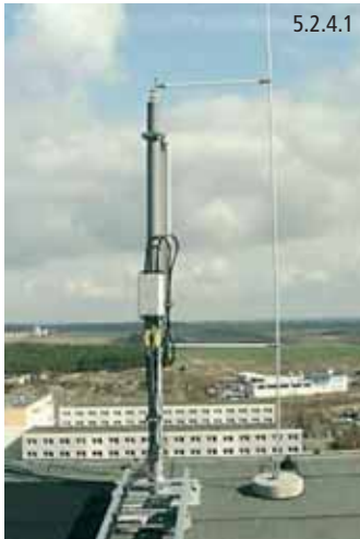
Fig. 5.2.4.1 Isolated air-termination system with distance holder
