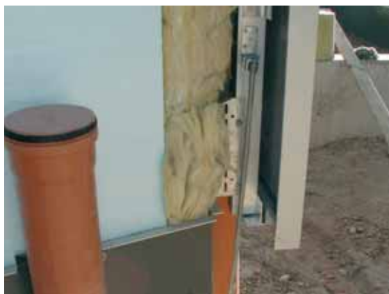
Fig. 5.2.2.2.3 Earth connection of a metal facade
