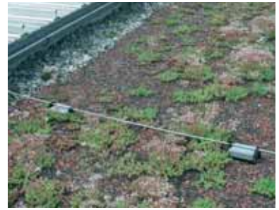
Fig. 5.1.7.3 Conductor leading on the covering layer
