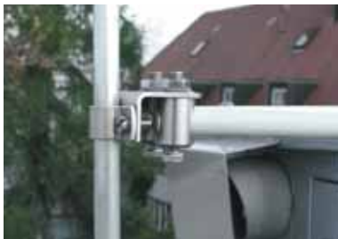
Fig. 5.1.8.5 Supporting element for the air-termination rod
