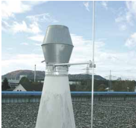
Fig. 5.1.8.3 Air-termination rod with distance holder
