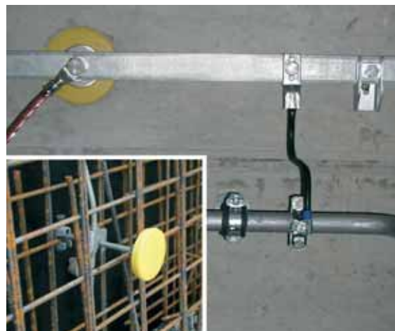
Fig. 5.5.2.8 Fixed earthing terminal
