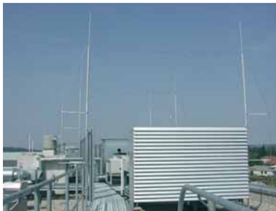
Fig. 5.1.8.12 Isolated air-termination systems with DEHNiso-Combi
