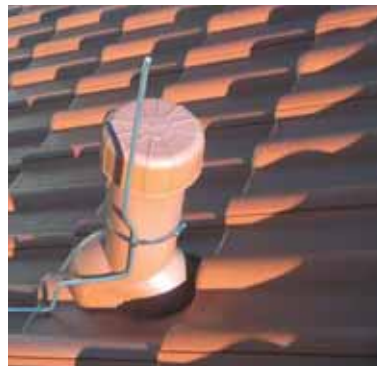
Fig. 5.1.2.3 Additional air-termination system for ventilation pipes
