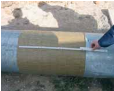
Fig. 5.1.8.8 Additional protection in the transition area by anticorrosive band for underground application
