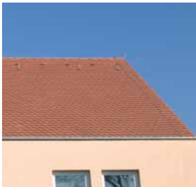
Fig. 5.1.2.1 Air-termination system on a gable roof
