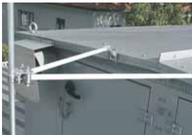
Fig. 5.1.8.4 Angled support for air-termination rods
