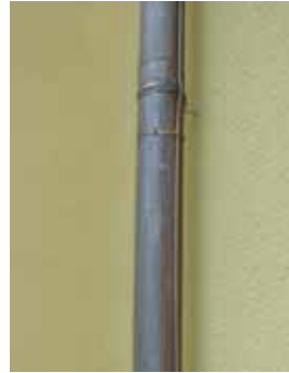
Fig. 5.2.2.2.4 Down conductor installed along a downpipe
