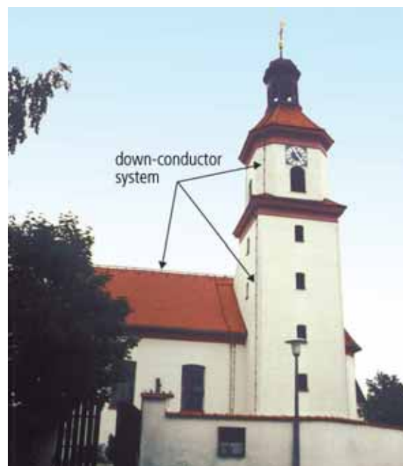
Fig. 5.1.9.1 Installing the down-conductor system at a steeple
