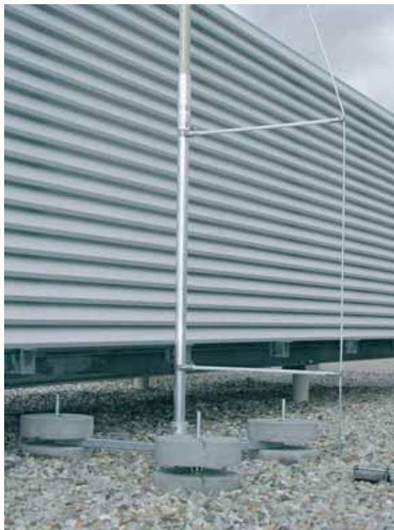
Fig. 5.1.8.11 Tripod support for self-supporting insulating pipes
