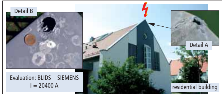
Fig. 5.1.4.2 Example of damage: Metal plate cover
