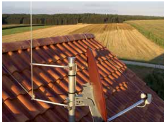
Fig. 5.1.2.5 Antenna with air-termination rod
