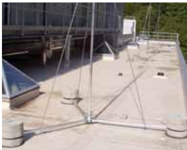
Fig. 5.1.8.7 Isolated air-termination system for roof-mounted structures
