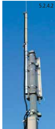
Fig. 5.2.4.1 Isolated air-termination system with distance holder
