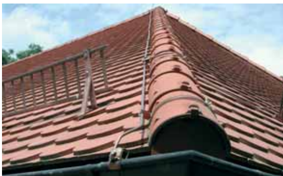
Fig. 5.1.1.18 Gable roof with conductor holder
