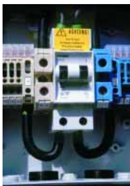
Figura 3.101 - Interruptor principal DC
